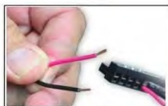
Strip each conductor 1/4"
