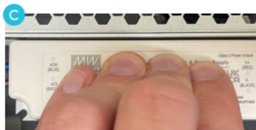
Install New Power Supply
