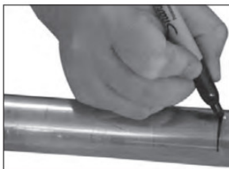
Figure 3 — Marking for Insertion Depth
