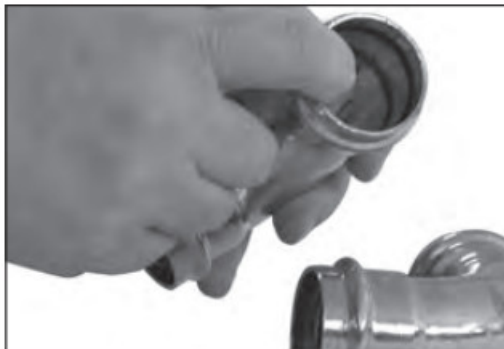
Figure 2 — Check for EPDM Seal
