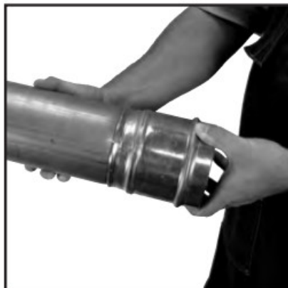
Figure 9: Inspection of final crimp
