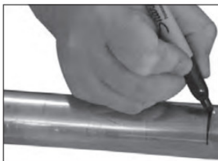
Figure 3 — Marking for Insertion Depth
