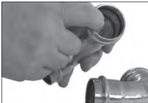
Figure 2 — Check for EPDM Seal
