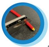
6 Cut off the end of the existing drain line to remove the old flow restrictor
