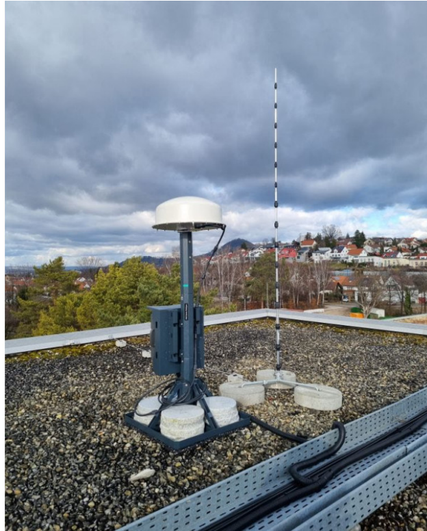
Figure 2: ADFA installation with optimized lightning conductor
