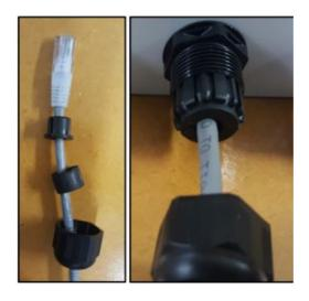
• Plug the RJ45 connector on the end of the (one to one) Ethernet (LAN) cable into the socket on the transmitter modules board. Allow the Ethernet (LAN) cable to take a gradual bend then tighten the compression nut onto the cable gland to form a weatherproof seal. See the image below.
