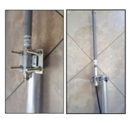
• Fit the washers provided with each U Bolt / Bolt and tighten the nuts accordingly without damaging the mounting pole.
