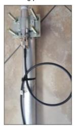
Referring to image above, connect the 1M RG58 antenna cable to the Antenna and loop the cable once (to allow for contraction and expansion) and fix the antenna cable to the post using a cable tie. Leave the other end of the cable loose for now.
