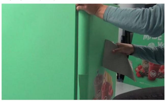
25. Spray panel surface with isopropyl alcohol, scrub surface with clean cloth to remove dirt or adhesive residue. Dry thoroughly with a different clean cloth. Make sure surface is dry and dirt/lint free.
