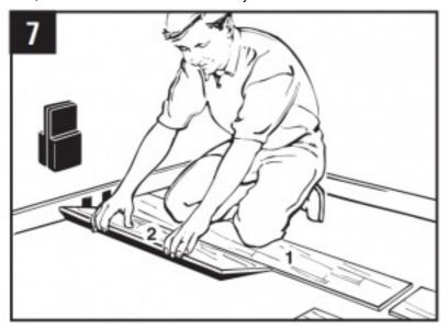
8. Join the short end of the plank first. There will be a gap on the long side joints when the plank is rotated down.
