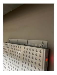
Next mark your holes on the wall and move the panel for drilling and installation of the anchors.
