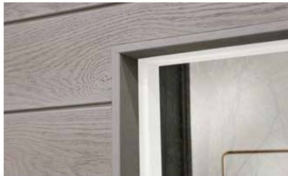
Fig. 14 - Window/door head with mitred joint
