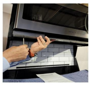
Step #4: Once the left screw is installed and the bracket is stable, insert the second adapter and screw in the samefashion. Do not fully tighten.
