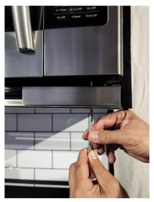
Step #5: Once both adapters are installed, and flush with outside edges of microwave unit frame tighten both screws until seated firmly. You do not need to over tighten, just make sure to tighten the screws firmly. Completed installation look/ see picture:
