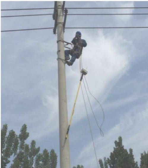
Figure 31: Lifting the equipment using a climbing equipment and a rope
