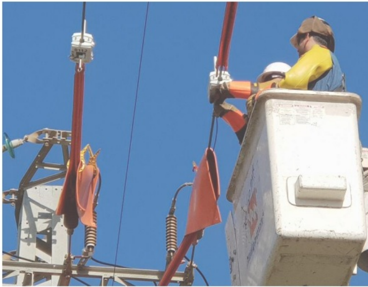
Figure 25: Direct Installation on a live line using insulated gloves and insulated aerial platform
