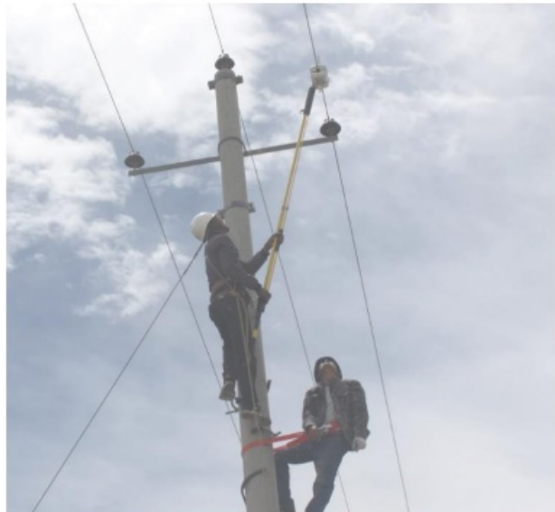
Figure 32: Installation by hot stick (fastening the secondary clamp screw)
