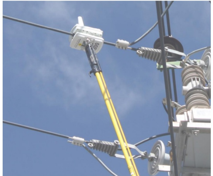
Figure 22: Fastening the main clamp screw
