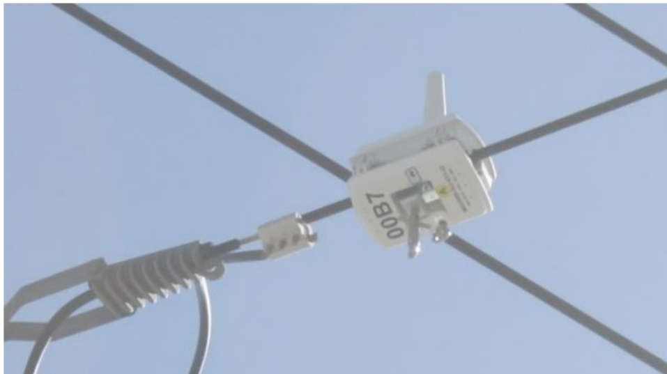
Figure 23: Sensor attached to wire but still open
