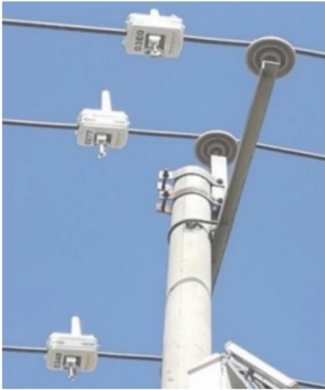
Figure 29: Sensor installed on each phase
