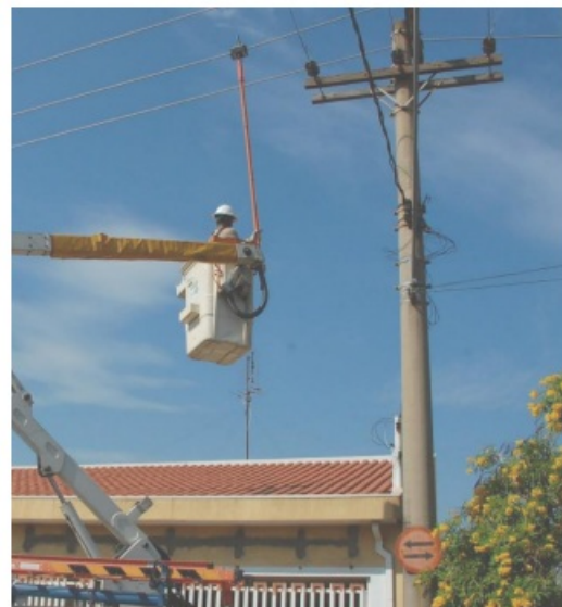
Figure 32: Installation by hot stick (fastening the secondary clamp screw)
