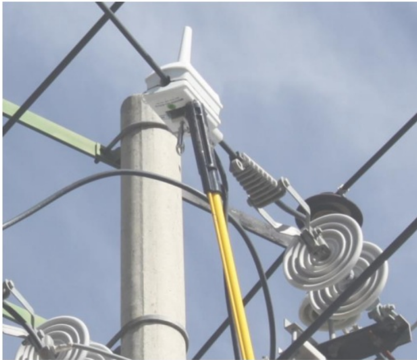
Figure 24: Fasten the secondary clamp screw
