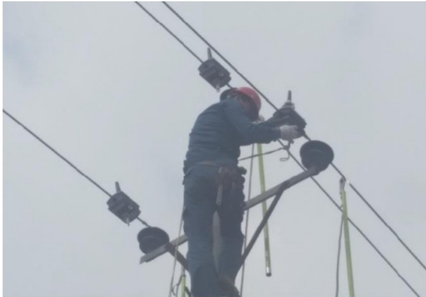
Figure 26: Direct installation on a non-energized line
