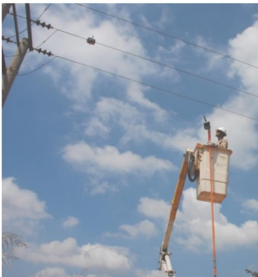
Figure 31: Lifting the equipment using a climbing equipment and a rope
