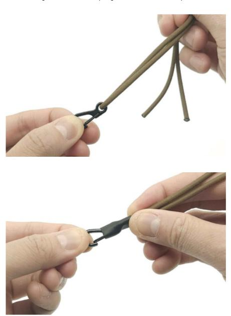
Secure the spring hooks using the provided heat shrinks.
