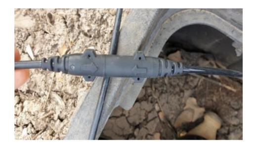
**Step 6)**Activate the Allegro Pit Unit using a magnet or Allegro Activator tool
