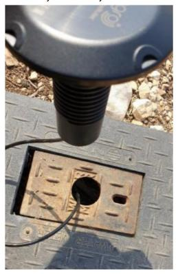
**Step 4)**Fasten the unit to the meter pit lid using the threaded locking mechanism
