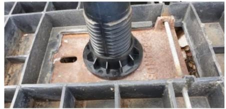
**Step 5)**Attach the Allegro Pit Unit to the encoded water meter using the appropriate Nicor or Bare Wire connections
