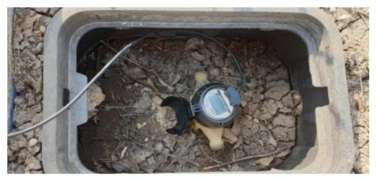
**Step 2)**Remove threaded locking mechanism
