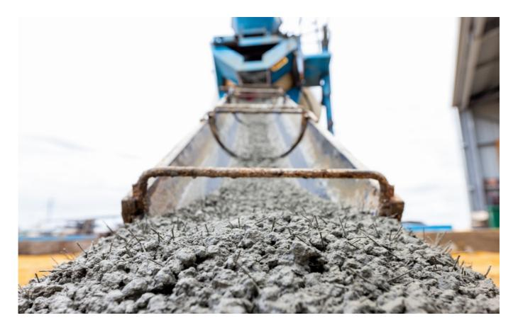
Polypropylene fiber for reinforcement in sprayed concrete and cast concrete applications as an alternative and/or supplement to existing concrete reinforcement products
