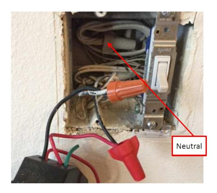
Connect wires according the marks on the switch.
