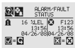
Figure 162. Alarm/Fault Status screen
