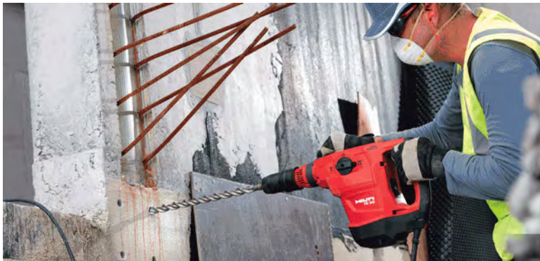
Fig. 9.4: Hammer drilling (HD) tools
