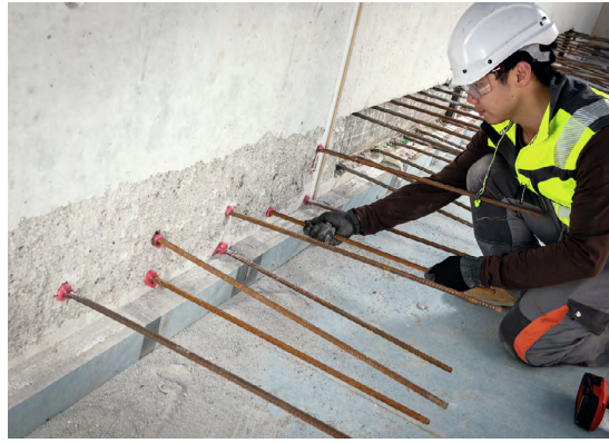
b) Slab-to-wall connection
