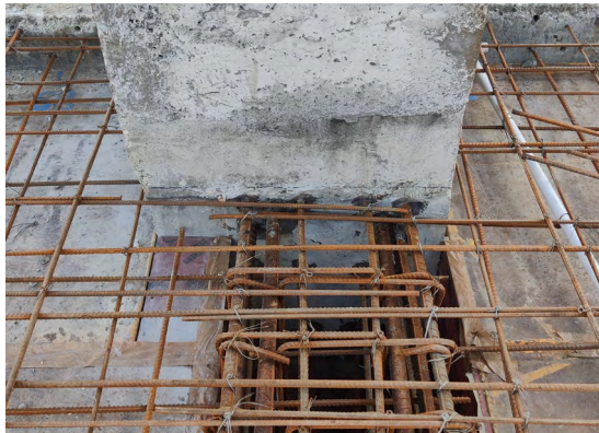
d) Beam-to-column connection
