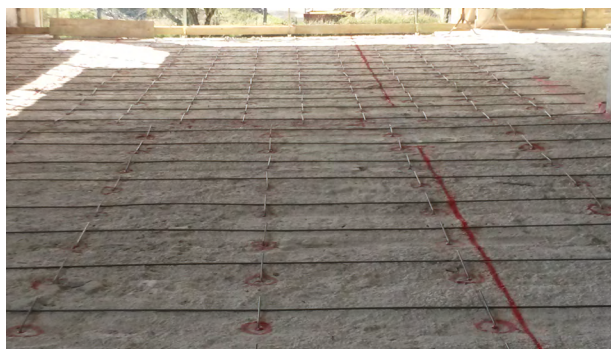
a) Concrete overlay on existing floors
