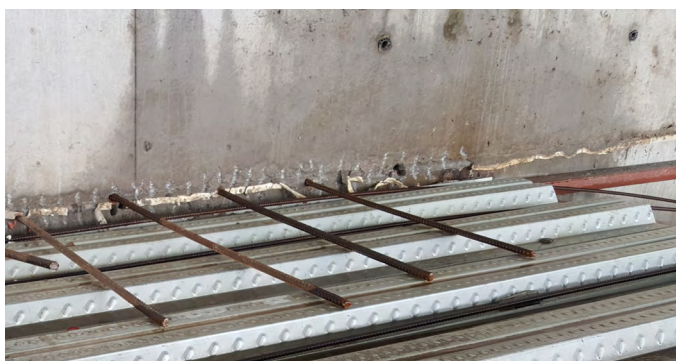
b) Post-installed rebars installation for slab to wall connection
