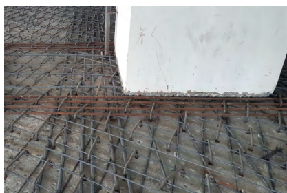
c) Slab strengthening
