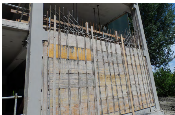
a) Corner walls
