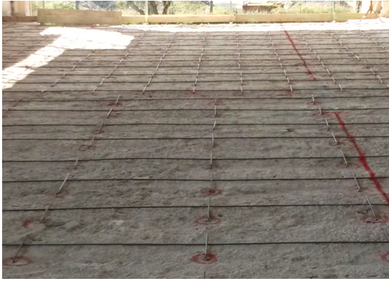
g) Slab shear-friction overlay
