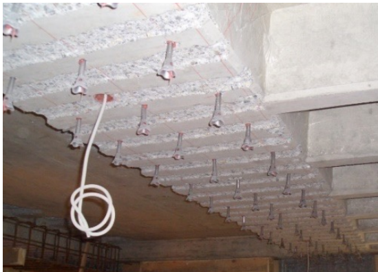
a) Increasing RC beam depth
