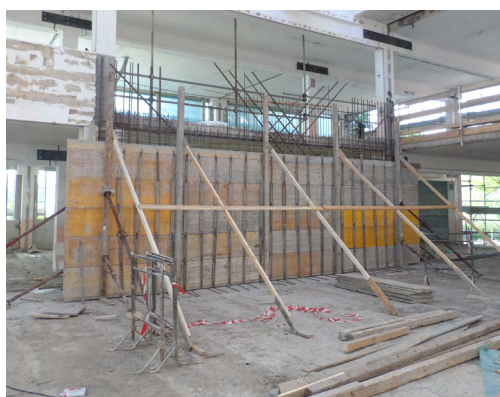
b) Interior walls
