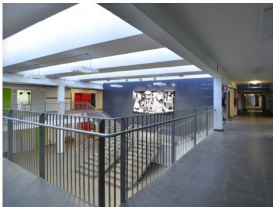
a) Building after seismic intervention
