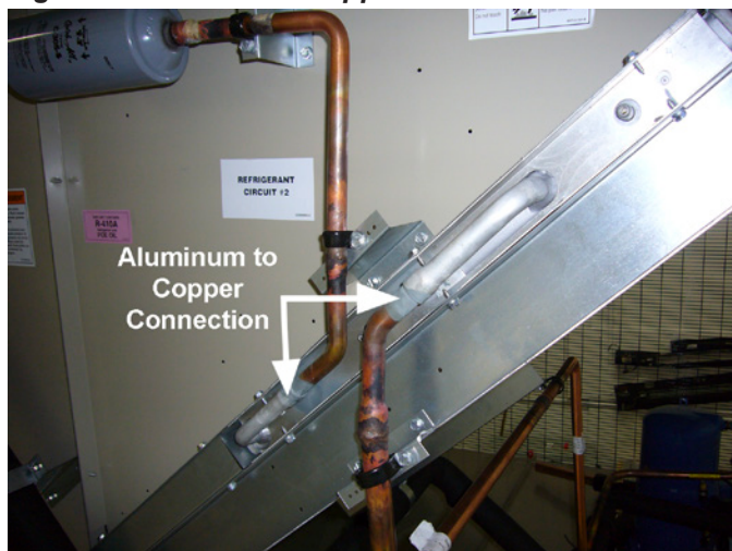
Figure 62: Aluminum/Copper Connection
