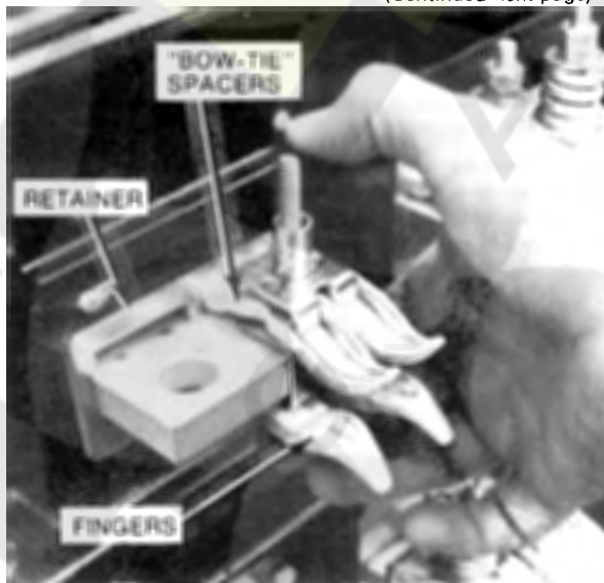
Fig. 45. Partial primary disconnect ASM
