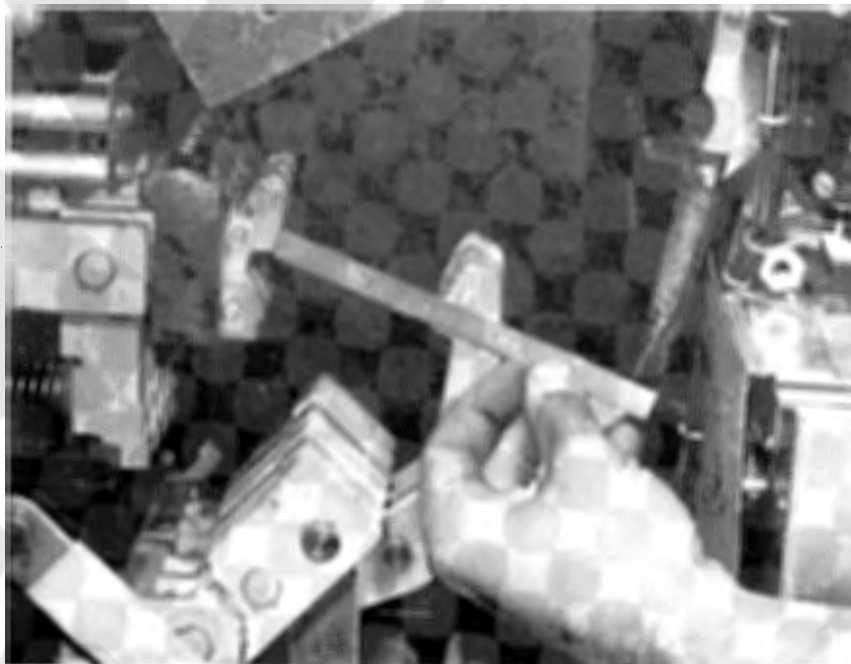
Fig. 13. Measuring contact open gap
