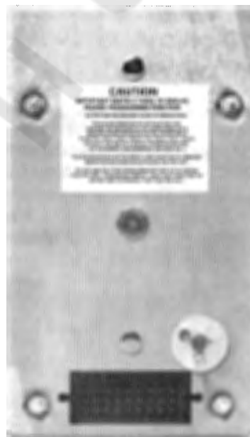
Fig. 113. Rear view of MicroVersaTrip PM Trip Unit.
