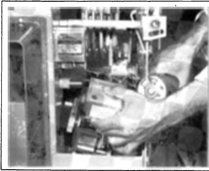
Fig. 32. Motor operator removal
