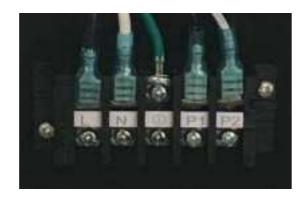
Position L,N and is for the power connection of our heat pump.
