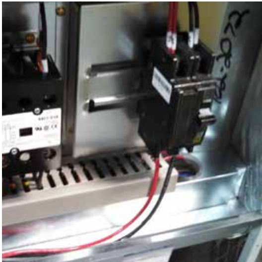
FIGURE 14 Wire Routing
