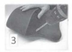
We don't pre-drill wire lead holes so you can put them where you want them. But a good place is the underside of each pod (image 2) so there will be no visible wires once installed. With a pod in place, little pieces of tape on the pod and the carpet can act as markers. Remove the pod, then use a 7/16" paddle bit and drill out the hole about an inch in from the edge (image 3). Repeat process in mirror image for other pod. Install the rubber grommets.
