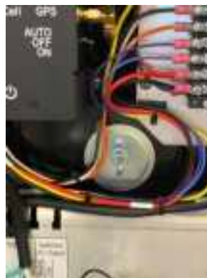
Hole Plug installed
