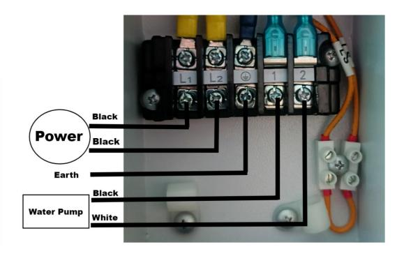
The output of the VDPYCA-110、VDPYCA-150、VDPYCA-210 pump terminal is
