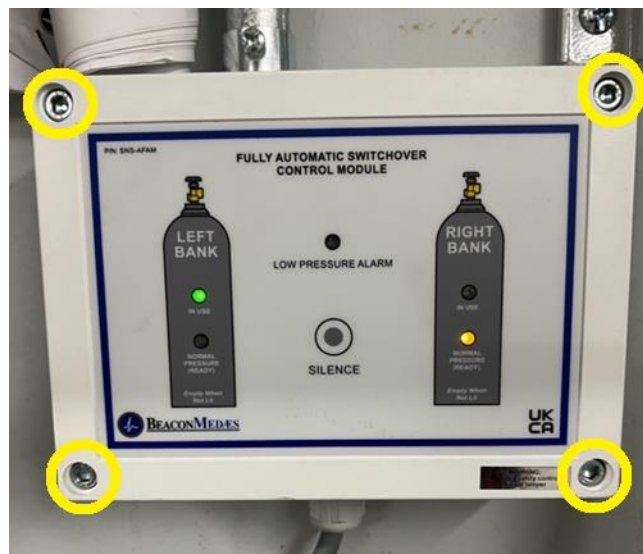
Figure 1: Four screws on the front cover of the Fully Automatic Switchover Control Module
