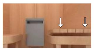
**Step 13: Guard Rail**Screw the guard rail pieces as shown and set the Guard Rail in front assembled to the Heater.
