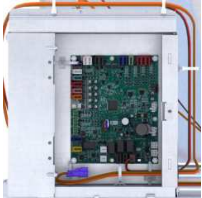
Figure 26. Power connection to return control box - all units
