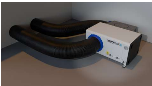
Surface mounted outside the growing area with plenumbox (check chapter 6.6 for connecting air hoses)
