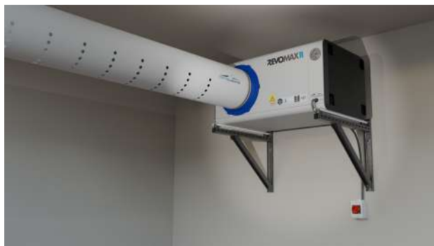
Wall mounted with airhose inside growing area
