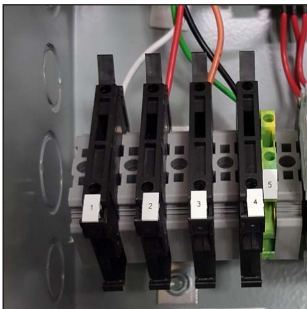
FIGURE 2 LC6000 Fused Power Supply Terminals
