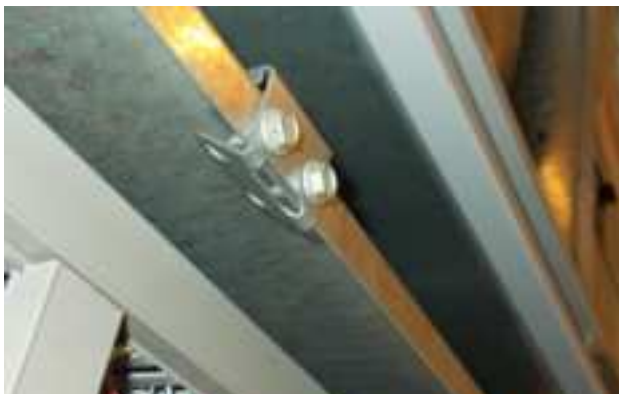
FIGURE 40 Re-Install Screws and Bend Tabs Up
