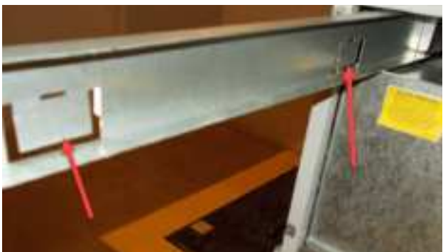
FIGURE 37 Bend Filter Tabs Down
