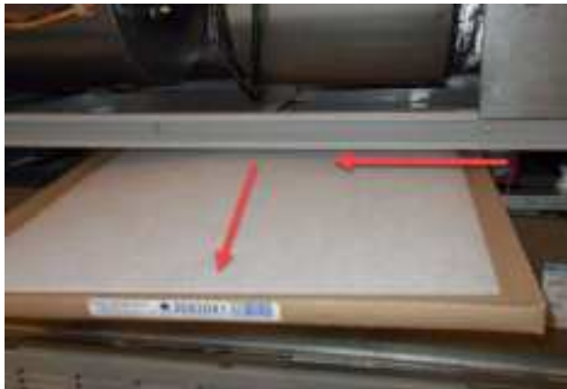
FIGURE 35 Removing Second Filter
