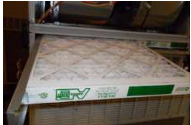
FIGURE 42 Install Left 2" Filter
