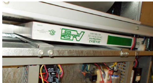
FIGURE 42 Install Left 2" Filter
