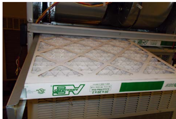
FIGURE 42 Install Left 2" Filter
