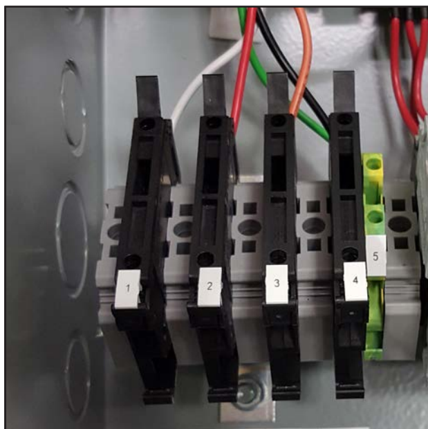
FIGURE 2 LC6000 Fused Power Supply Terminals
