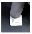
Note: Paste the Cable tie bases and insert the cable ties after following the cleaning & primer application process, reference location for 25 pasting the tie base is in step 27.
