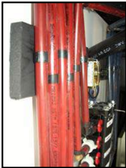
Figure 11-10. Plumbing Manifold
