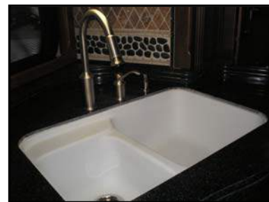
Figure 11-2. Kitchen Sink & Counter
