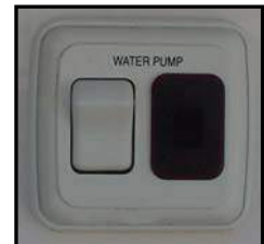
Figure 11-6. Water Pump Switch
