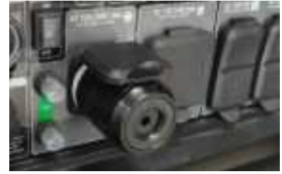
NEMA L14-30P Bonding Plug
