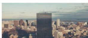
Heating & Air Conditioning
