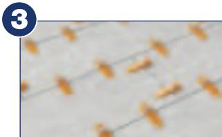
3 Slide wedges into clips to level, align, space and hold the tiles
