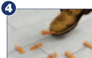
4 Once the mortar sets, break-off in direction of grout line within 24 hours
