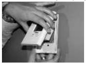
Align and secure the mounting base to the connection box using the two screws supplied;
