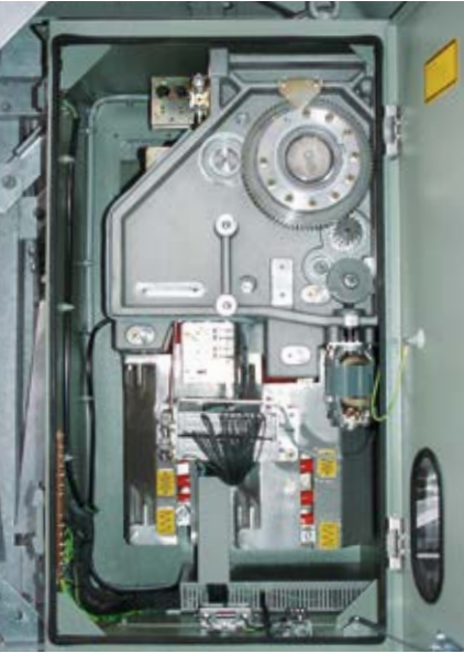
Control cubicle with circuit-breaker operating mechanism
