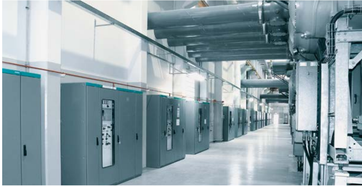
Control cubicle with circuit-breaker operating mechanism
