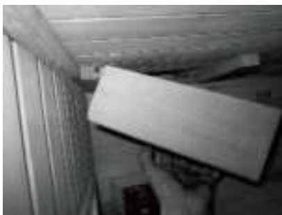
FIG 15.2 Installing the Radio Wood Housing
