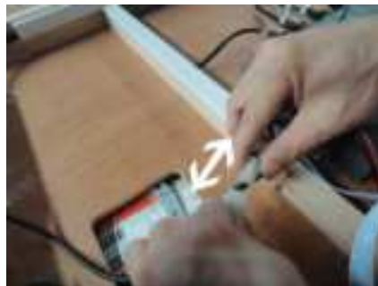
FIG 15.1 Screw CD Player into sauna room
