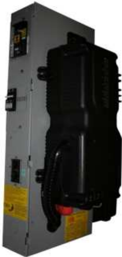
E-PANEL FOR MAGNUM MM SERIES AS INSTALLED
