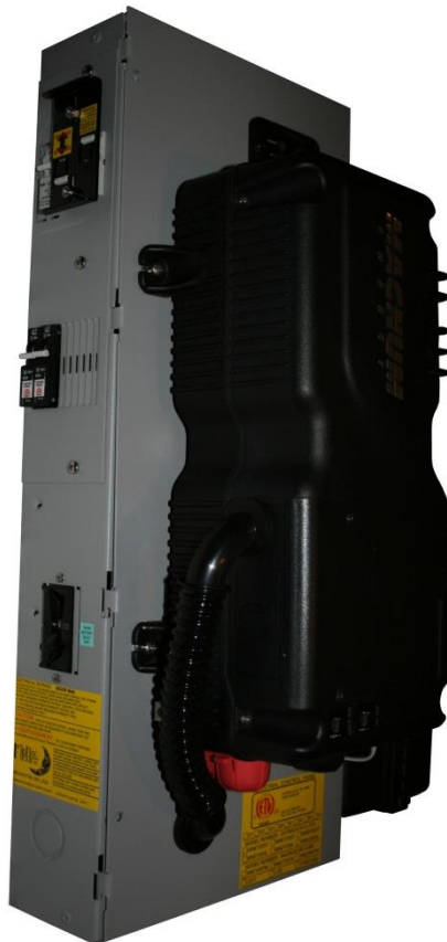
E-PANEL FOR MAGNUM MM SERIES AS INSTALLED
