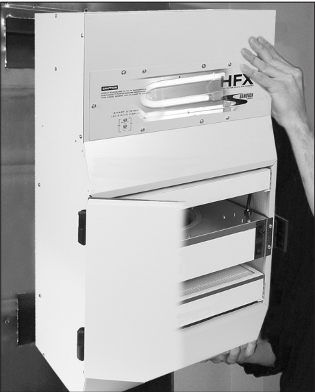
Figure 2.3a - Align unit into place.
