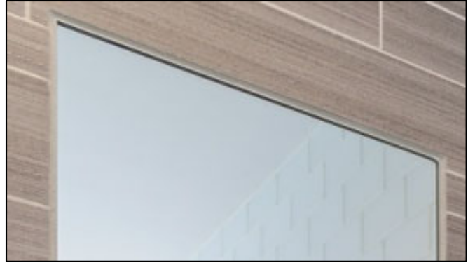
Figure 3. Grout around the mirror to seal and finish.
