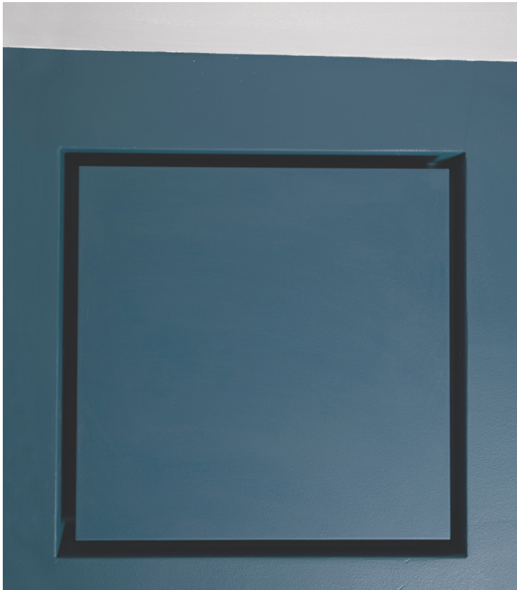
Above: bottom view of painted finish, installed Drywall Pro X. Center piece can be removed to access ventilation motor
