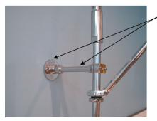
Cut the riser support rods to the proper length and attach flanges to the wall. IMPORTANT: INSTALLER IS RESPONSIBLE FOR ALL PLUMBING TO CONFORM TO LOCAL BUILDING CODES WHICH MAY BE DIFFERENT FROM ILLUSTRATIONS SHOWN IN THIS MANUAL.
