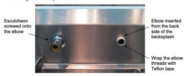
Loosely fit the escutcheons to the elbows and the faucet body. When the alignment of the body with the sink is confirmed, tighten the escutcheons onto the elbows and faucet body. From the back side of the backsplash, tighten the brass nuts on the elbows when the faucet body is parallel with the rim of the sink.
