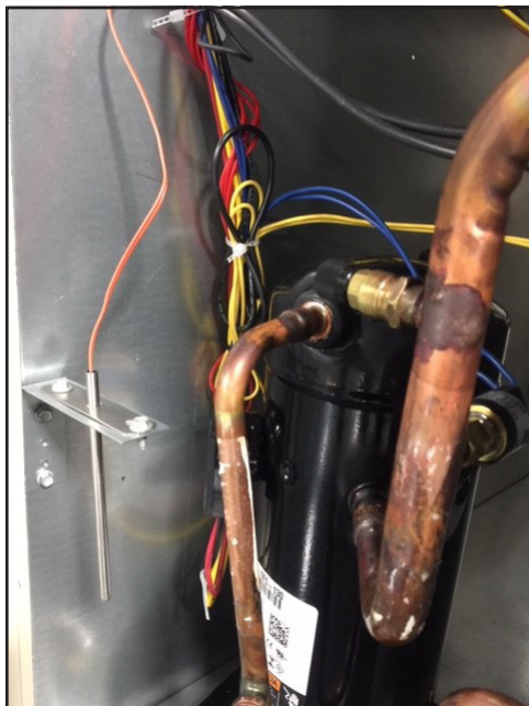
FIGURE 6 Outdoor Air Sensor Installation
